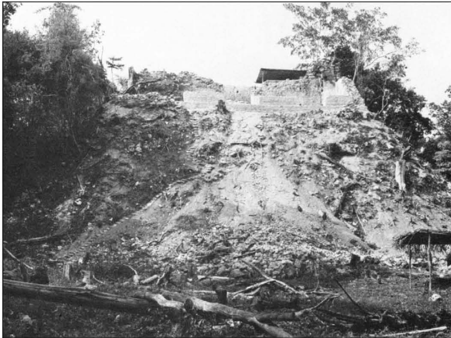
Fig. 6 Caracol Structure A3 during consolidation.
