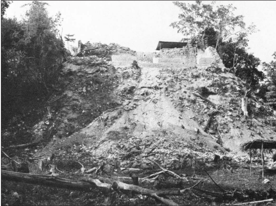
Fig. 6 Caracol Structure A3 during consolidation.
