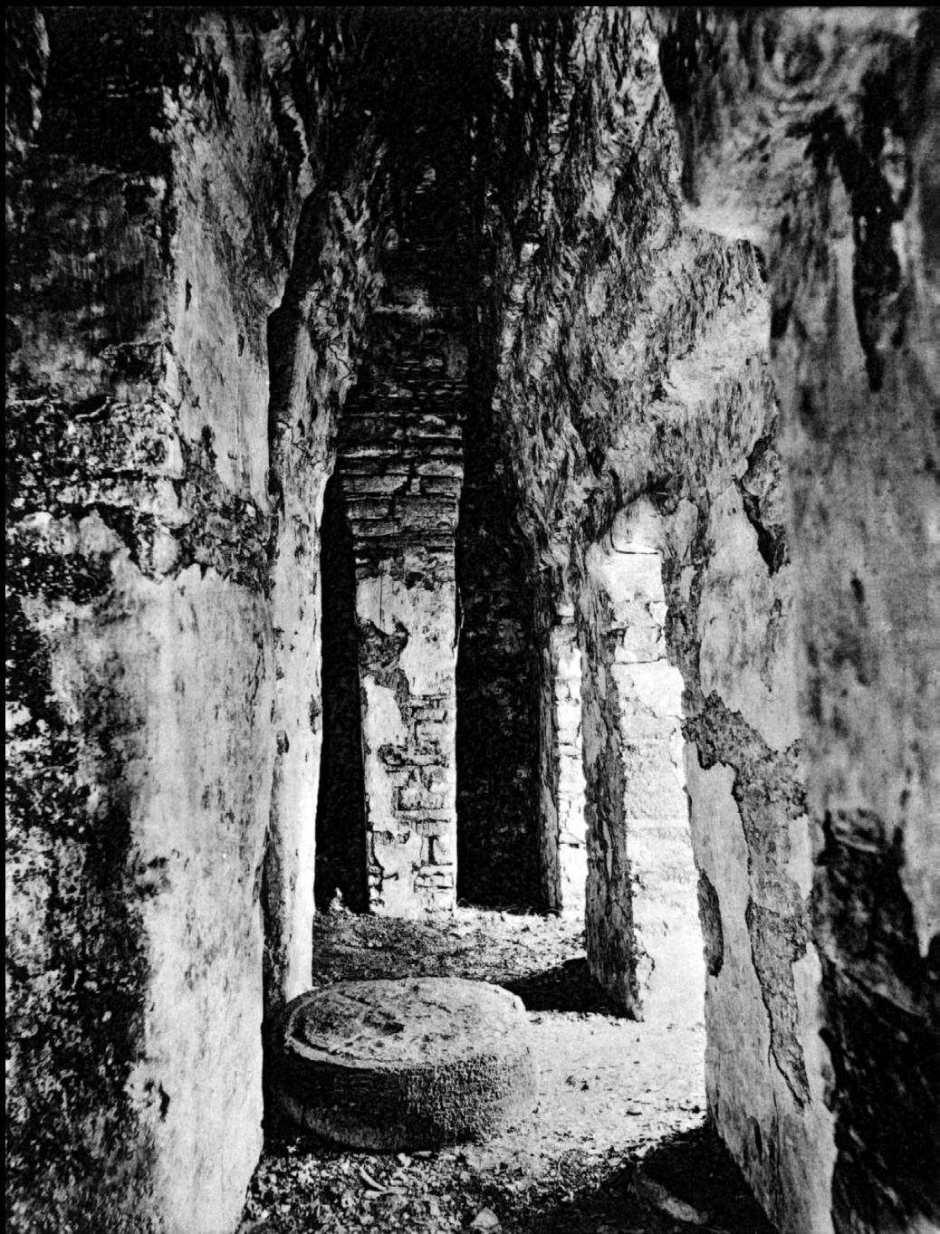
Yaxchilan: Interior Structure 39. After Maler 1903: Plate XLV, 2.
