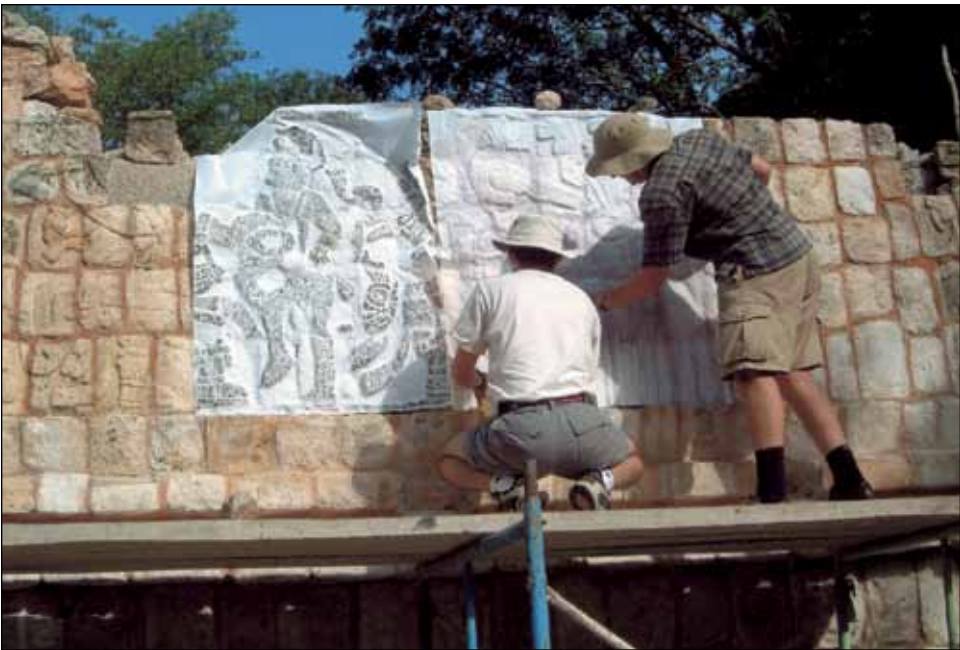
Applying the paper on the Casa de los Monos
